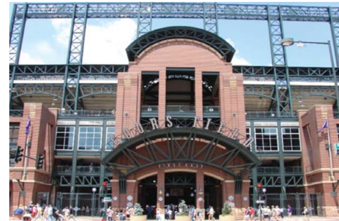
Coors Field Exterior
